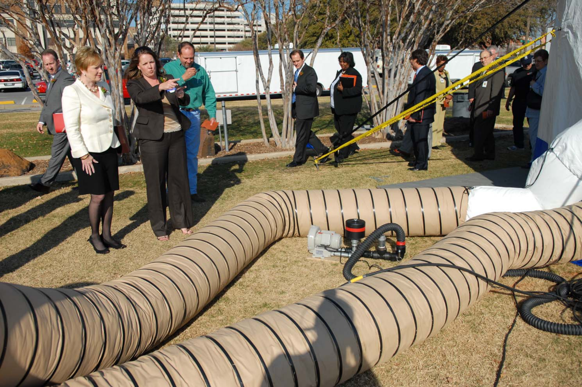
Insulated ducts to 5 ton HVAC unit with heat
