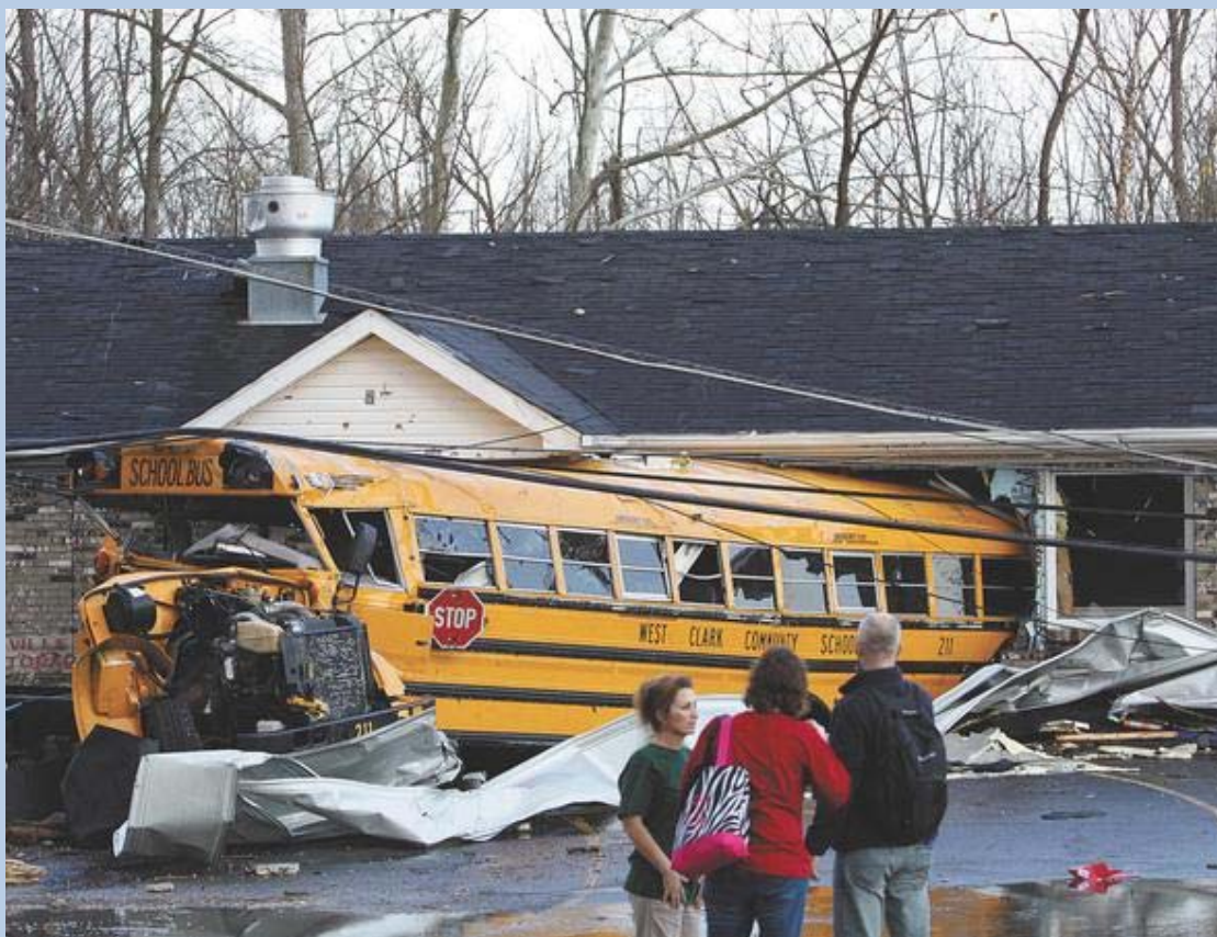
School bus pushed into a local diner in Henryville
