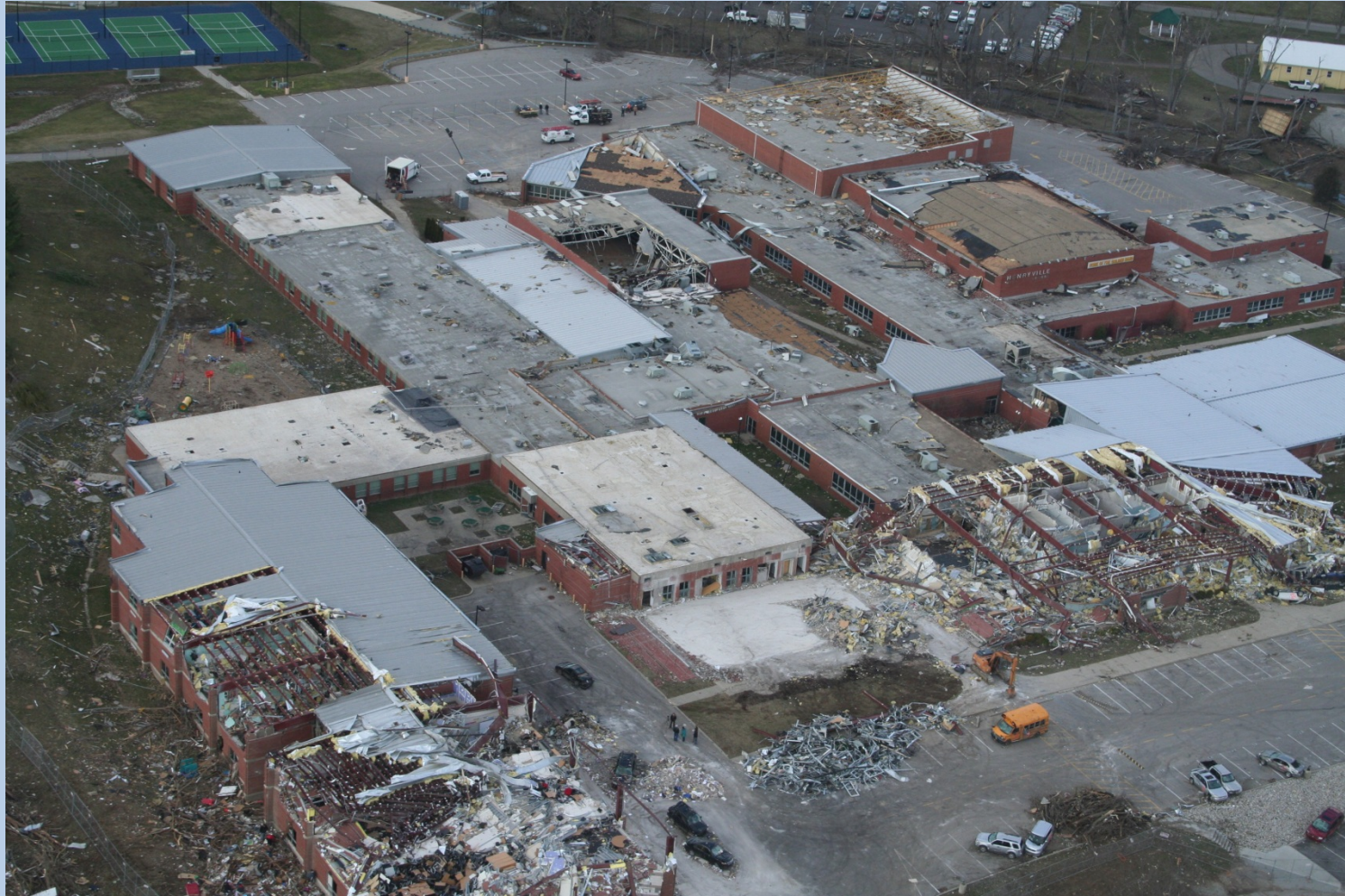
Henryville High School Complex – Received brunt of EF-4 damage
