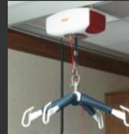
Ceiling lifts in patient rooms
